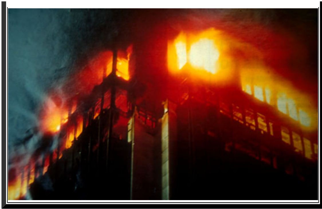
First interstate Bank Building (Los Angeles) Fire resistive type construction (believe it or not!) Photo by: New York Board of Underwriters
