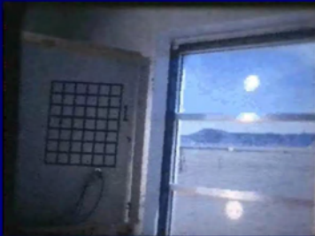
Deployable Catcher Bars Behind Window with 7 mil Daylight Film
